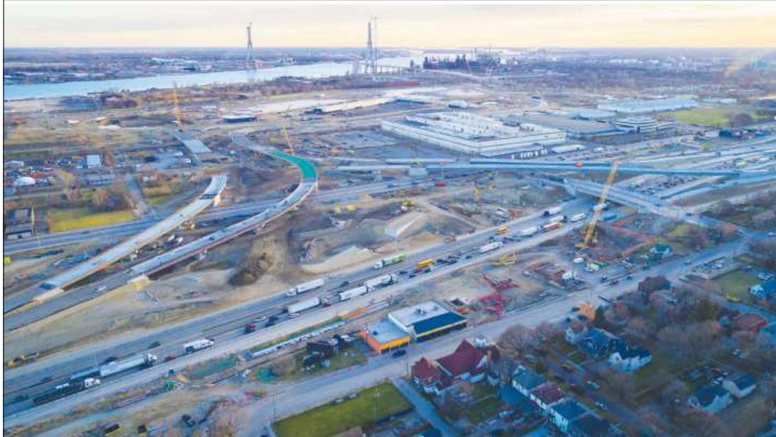
THE $4.8 BILLION price tag on the Gordie Howe Bridge includes a massive change in the landscape "behind the bridge" on 167 acres in Southwest Detroit. The U.S. Point of Entry will have 13 buildings and include border inspection facilities for both passenger and commercial vehicles, control booths, and parking. Once constructed, this port will be one of the largest ports of entry in North America. Local road improvements include widening of I-75 and reconfiguration of ramps and service drives, as well as construction of four new road bridges, five new pedestrian bridges, and connecting ramps to and from the U.S. Point of Entry. The bridge will have a direct link to I-75.
