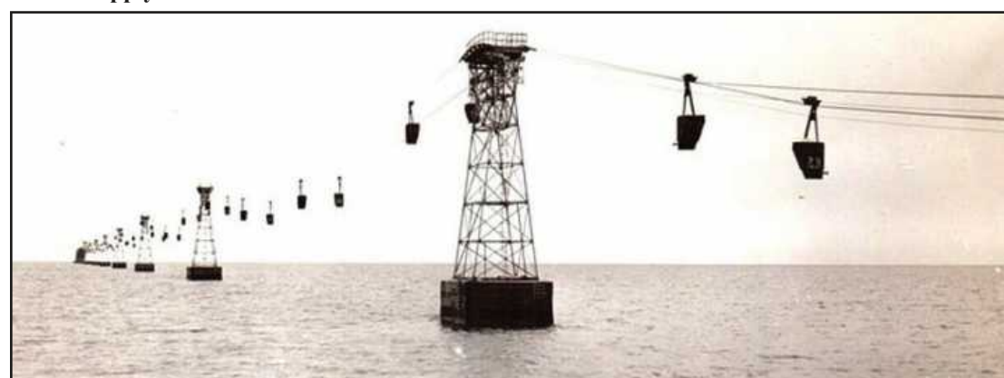
THE 400-ACRE ALABASTER Historic District was placed on the National Register of Historic Places, but there isn’t much still standing. “The most visible and impressive structure in the district, the elevated marine tramway, was constructed in 1928 and the tramway stretched 1.3 miles out into the Saginaw Bay,” says Lost in Michigan . “Like a horizontal ski-lift, the cable system carried 72 “buckets” of gypsum to a waiting ship or to the storage bin. Each bucket held more than two tons. The tramway included 6,450 feet of one- and three-quarter inch steel cable and 14,000 feet of three-quarter-inch cable. At a length of 6,350 feet, it was the longest over-water bucket tramway in the world.” The tramway was demolished in the 1990s and the loading marine bin in Lake Huron was finally torn down in 2020. This photo is from the 1940s.
