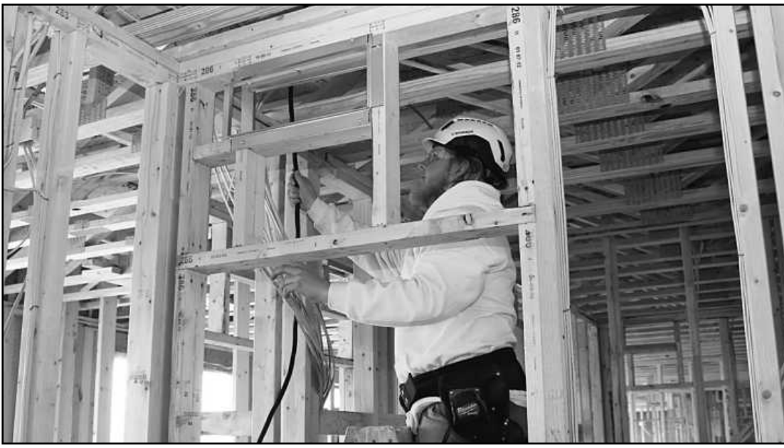
PULLING RANGE CABLE on the third floor of the Harrison Street Commons project in Flint is Max Hendrickson of IBEW Local 948. He is employed by Roth Electric.
